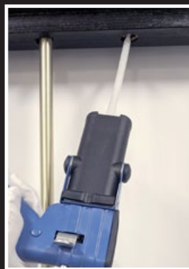
4. Epoxy handrail and cap/tread
