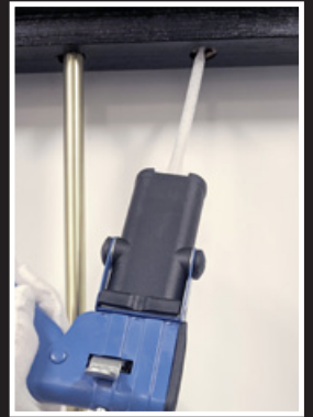
4. Epoxy handrail and cap/tread
