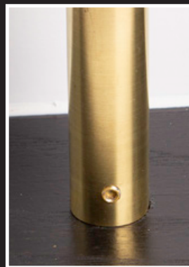
11. Sleeves are now in place, rotate balusters into position so set screws are facing desired direction before epoxy cures
